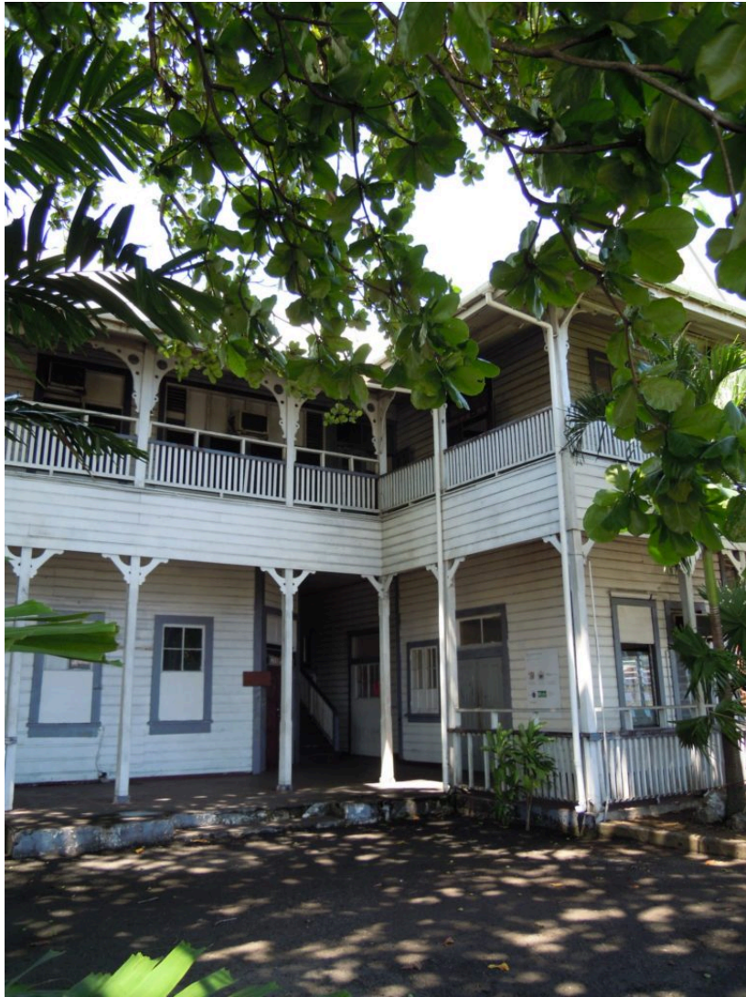
The former Apia Courthouse, built by the German colonial administration in 1902, © Julia Hütten
